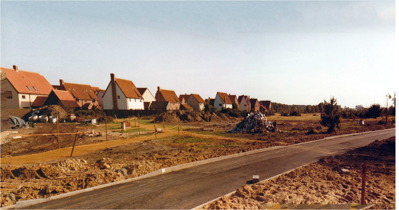
Back of Westland, looking south.
